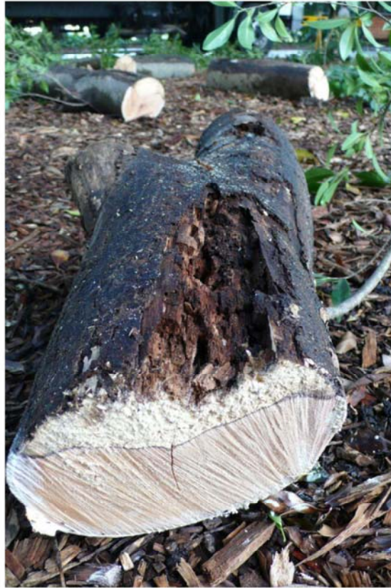
Photo C: Typical sunscald damage showing advanced wood decay and associated structural defect (Tree 242N).
